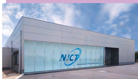
Kobe Clean Room
