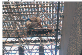
Figure 2 ● Fixing a supporting point of a Foucault pendulum Expert Jun-ichi Komuro at work
