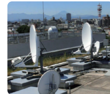
衛星時刻比較用アンテナ Antennas for time and frequency transfer via satellites
