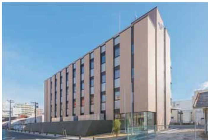
External appearance of Resilient ICT Research Center
