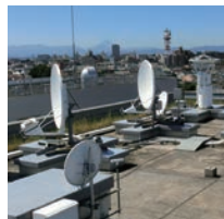
Satellite receiver antennas
