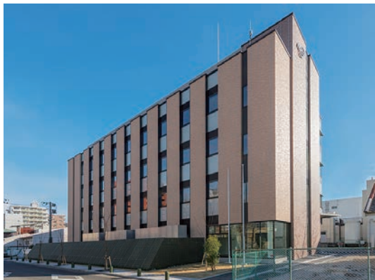
Resilient ICT Research Center (Tohoku University, Katahira Campus)
