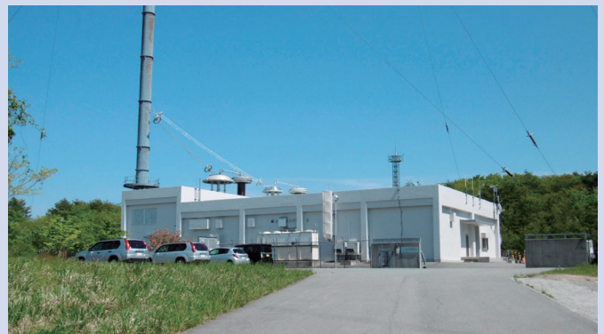
▲Standard time and frequency transmission station
