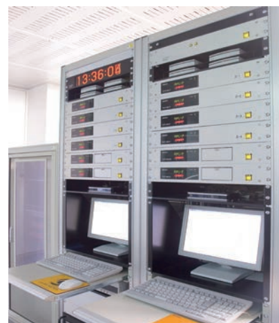
Telephone JJY System
