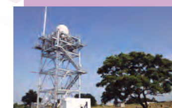
PANDA tower and container installed at the Advanced ICT Research Institute
