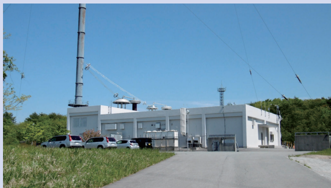
▲ Standard time and frequency transmission station
