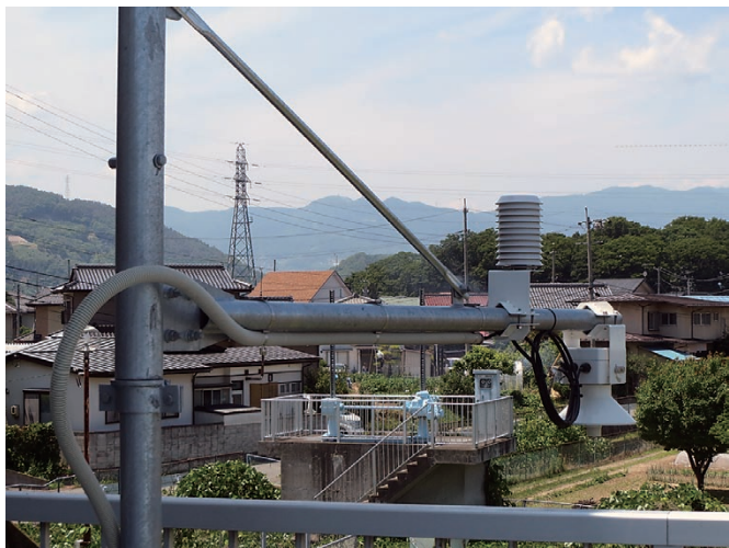
Figure 4 Water level sensor installed in the Sawayamagawa River basin
