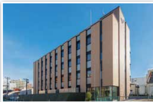
Resilient ICT Research Center, located in the Katahira Campus of Tohoku University
