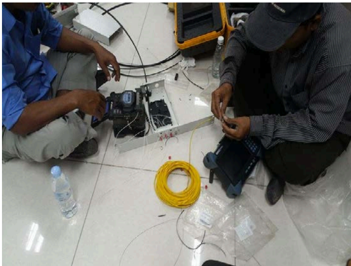
Connecting fiber optic from TC skun to Tower smart spun
