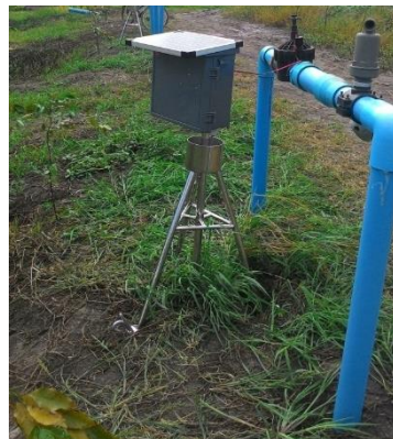
Valve Control Node
