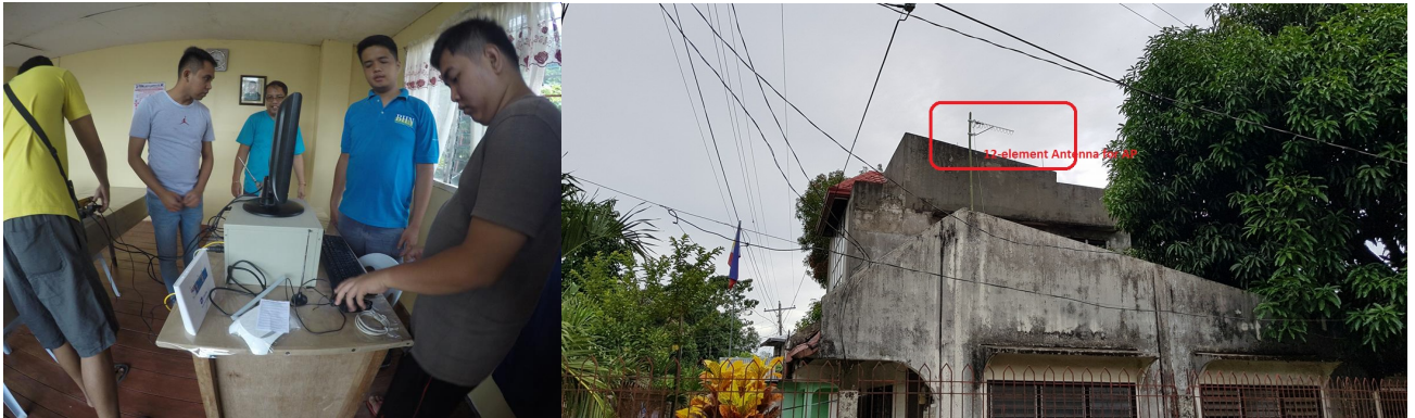
Figure 23. Configuring the AP inside the Bgy. Hall and placement of the 12-element antenna at the floor just outside where the team has installed the AP.
