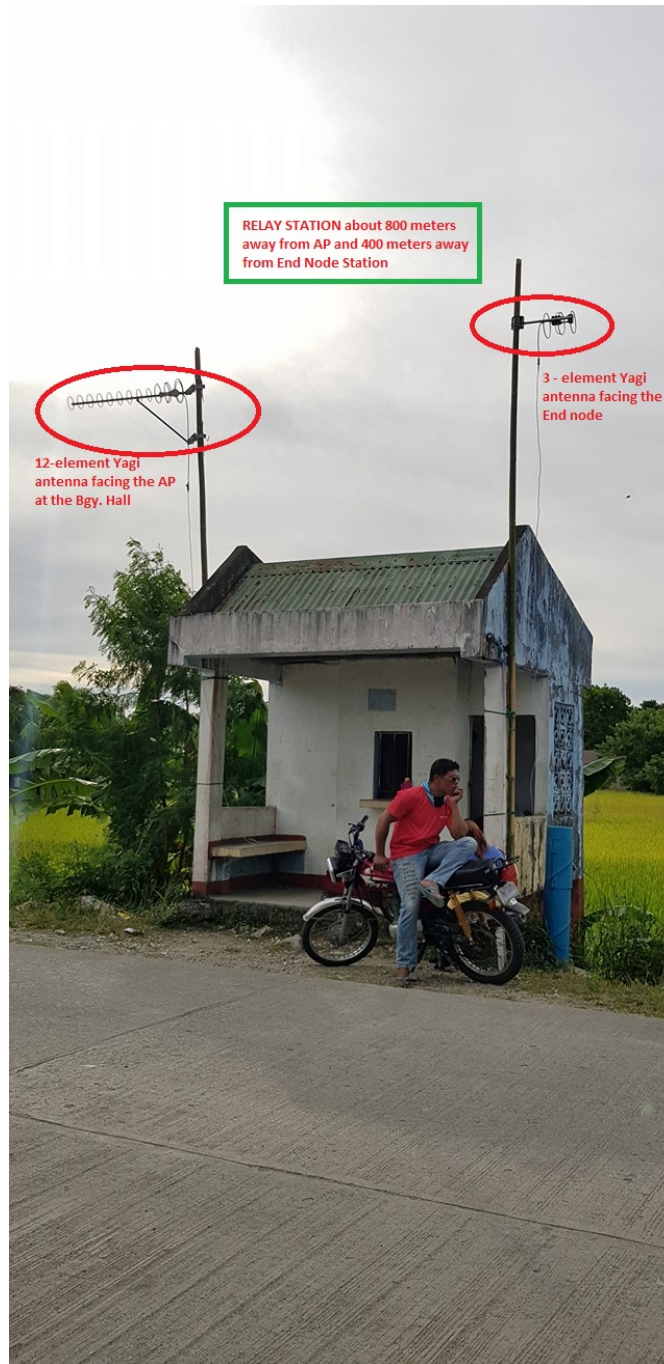
Figure 30. Relay Station about 800 meters away from AP and about 400 m away from End Node
