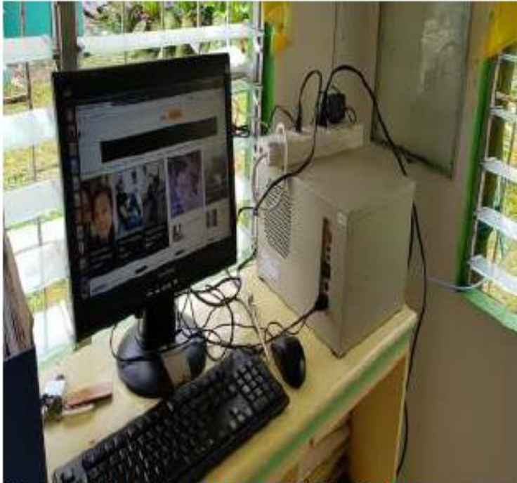
Figure Showing connectivity between AP (Bgy. Hall) and STA1 (Principal's Office)
